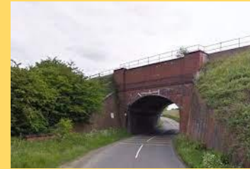
Westhouses railway bridge
